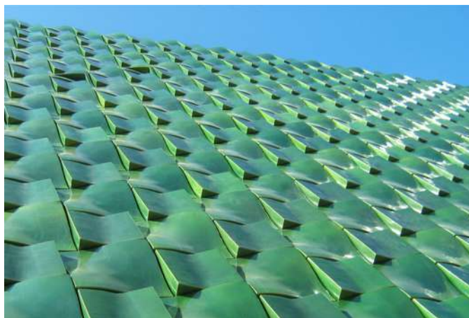
Figure 4 The ringling museum of art's facade shows us how digitally fabricated ceramic componentry can operate in conjunction with responsive custom glazes. Facade designed by Machado Silvetti Associates and Boston Valley Terra Cotta (see online version for colours)
